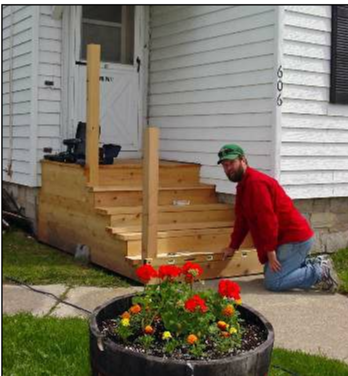
Replacing the rotten steps which leads up to the front door
