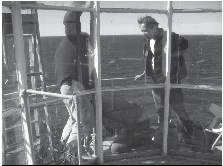
Peter Blanken (left) Mark Siegman (center) and Pakorn Petchprayoon (right) insert the mast into its flange on a custom cut plywood base on the narrow lantern gallery
