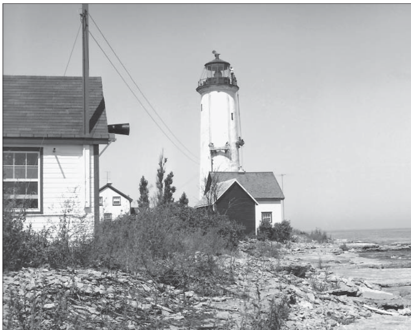
The fog signal building and tower at False Duck Island light station ca. 1960
