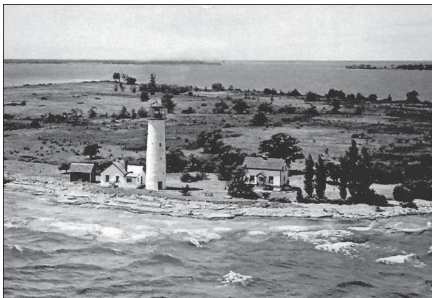
An undated photograph showing False Duck Island light station from the air.
