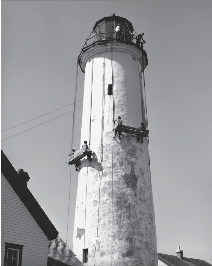
Painting the tower at False Duck Island at some the in the early 1960's
