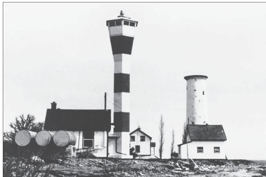
Both towers still standing before the old tower was demolished in June 1966
