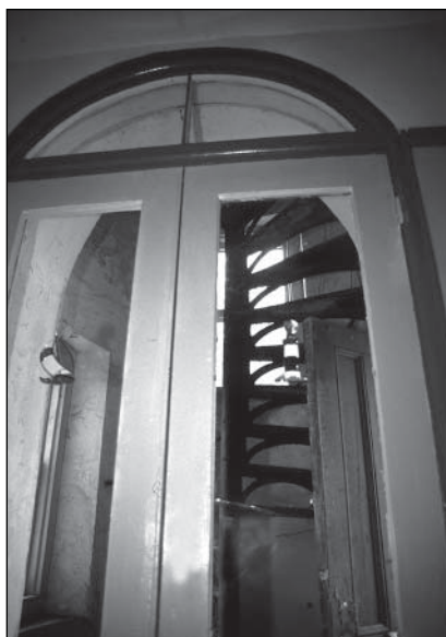
The unique double glass doors which lead from the dwelling into the tower
