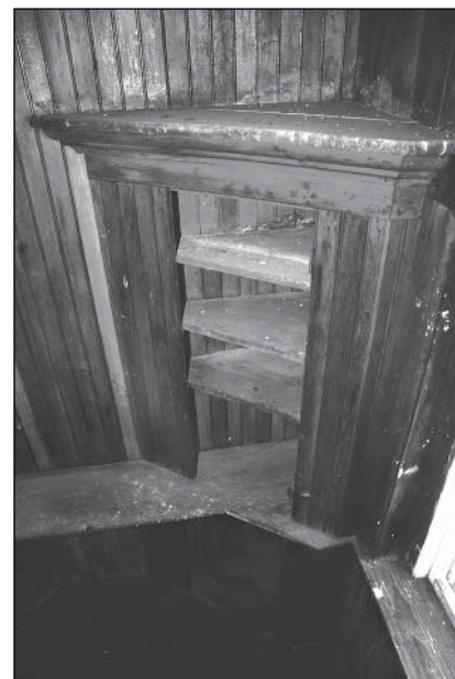
Corner supply cabinet in the watchroom The Beacon, Fall 2009
